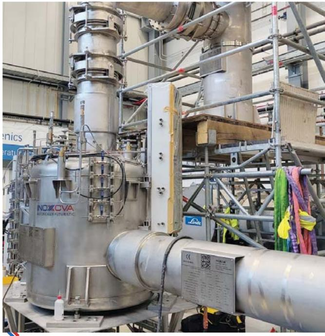
Installed image of Feedbox, Jumper and Transferline at FAIR Project
