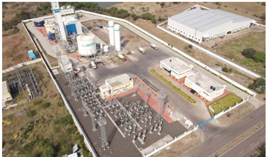
Installation of complete N2 package at Thailand 150kl + 8 vaporisers
