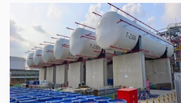
Hydrogen tank installation
