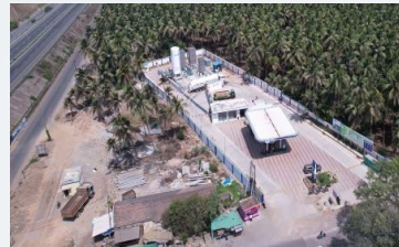
LNG/LCNG fuel stations
